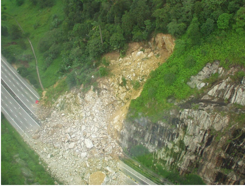
Landslide at Bukit Lanjan interchange North-South Expressway
