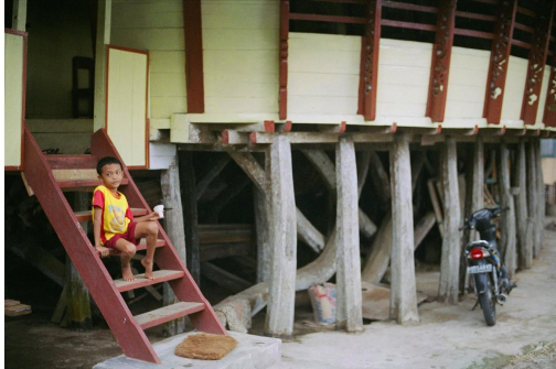
Traditional house with bracing for earthquake resistance
